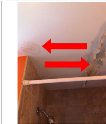
Water damage and staining
